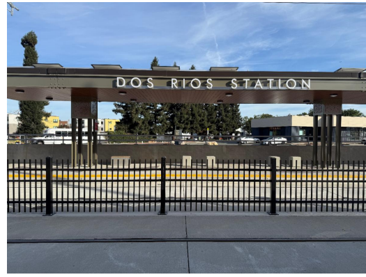
Platform fence at the New Dos Rios Station
