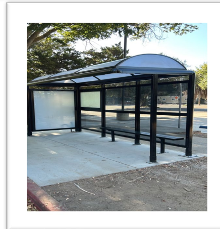
7 th & Q-Bus Stop Reinstalled
