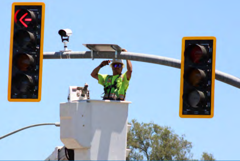
SIGNAL WORK AT 49TH STREET AND BROADWAY
