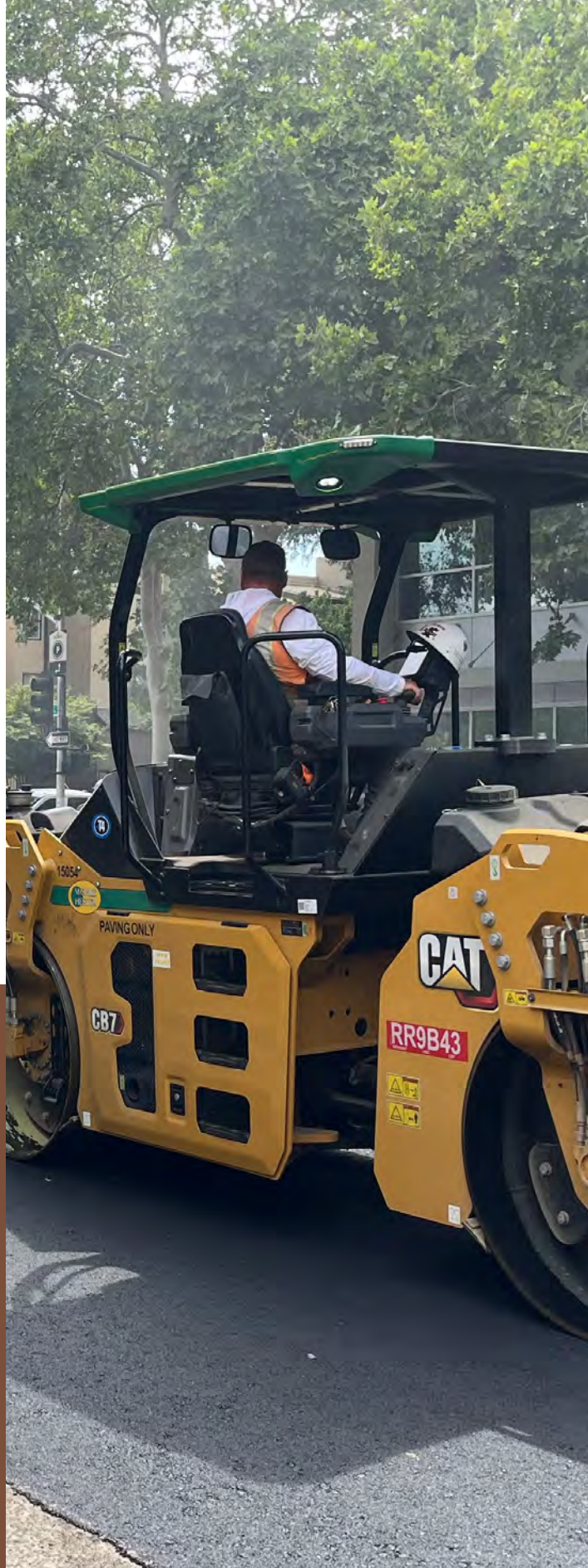
REPAVING ON 19TH ST
