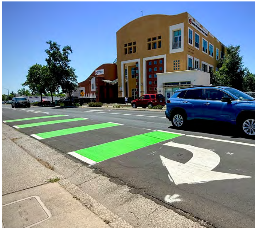
SAFETY PROJECT CONSTRUCTION ON MARYSVILLE BOULEVARD
