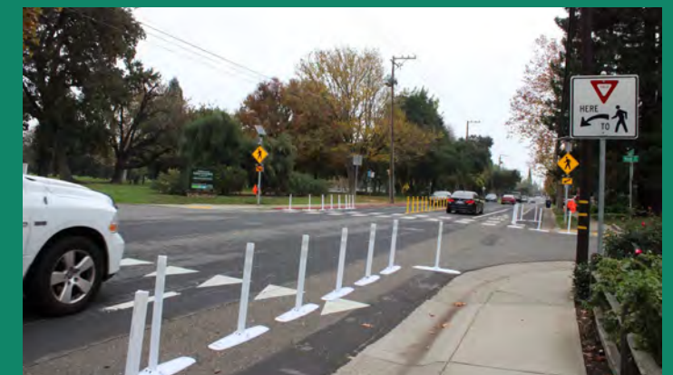
SUTTERVILLE ROAD QUICK-BUILD
