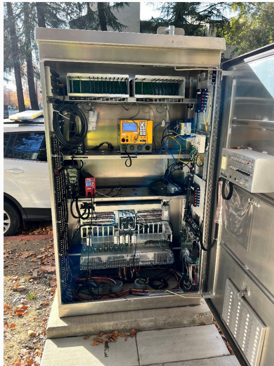
Traffic signal cabinet with new APS control unit
