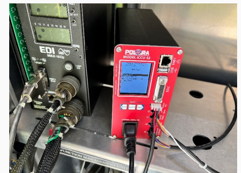
New APS control unit in cabinet
