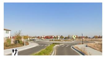
Mini Roundabouts / Traffic Circles: An unsignalized, circular intersection where incoming traffic yields to traffic in the intersection. Traffic circles require less space and may be stop controlled.
