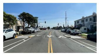
Pinch Point: Horizontal extension of the curb into the street, narrowing travel lanes by 1 to 2 feet requiring drivers to yield to each other.
