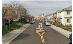
Median Islands provide a protected space placed in the center of the street to facilitate pedestrian and bicycle crossings.
